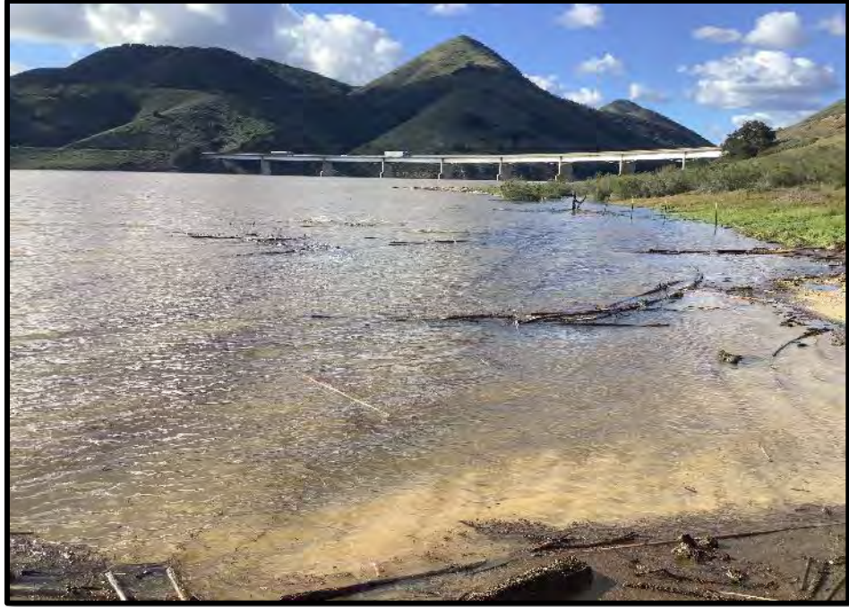
Figure 24. View of recently flooded docking area.
