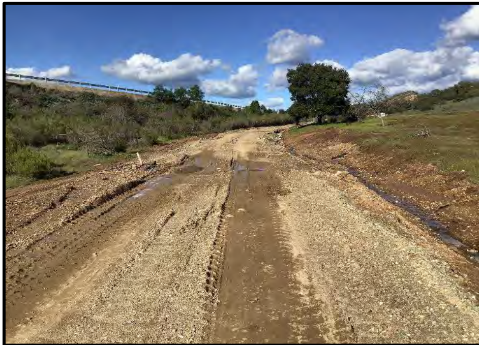
Figure 11. View of access road, taken approximately half-way to southern proposed stockpile location, facing northeast.
