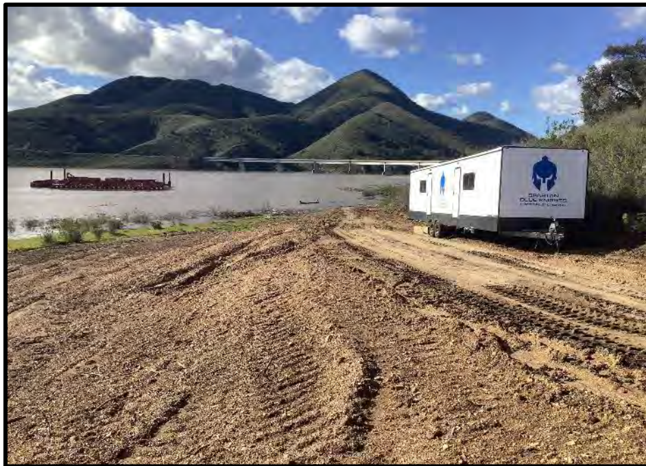
Figure 23. View of access road, emergency trailer, and barge. Taken from bend in access road, facing northwest.
